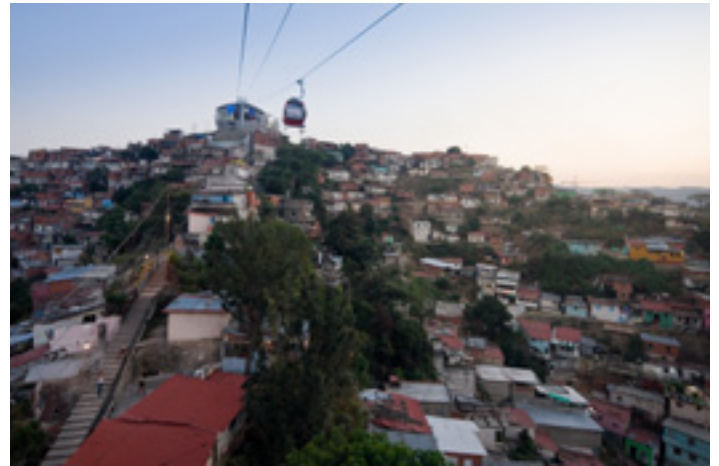
Urban Think Tank MetroCable project, Caracas, Venezuela (Photo: Iwan Baan)
