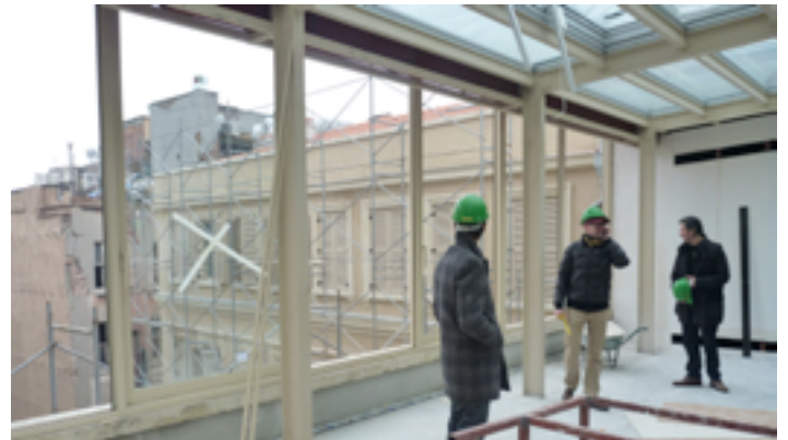
Garden at SALT Beyoğlu under construction
